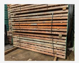
Soldiers (pictured on the left) are stacked together in four rows of five soldiers, regardless of size. Ply rips must be placed between each row with timber bites placed between each pack. All other accessories are placed into bins.
